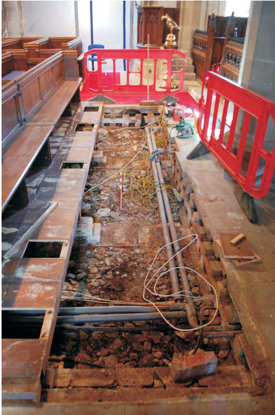
Plate 11. Interior view of Area B in St Mary's Church, Frittenden showing brick dwarf walls to support timber pew floor and recent rubble infill.
