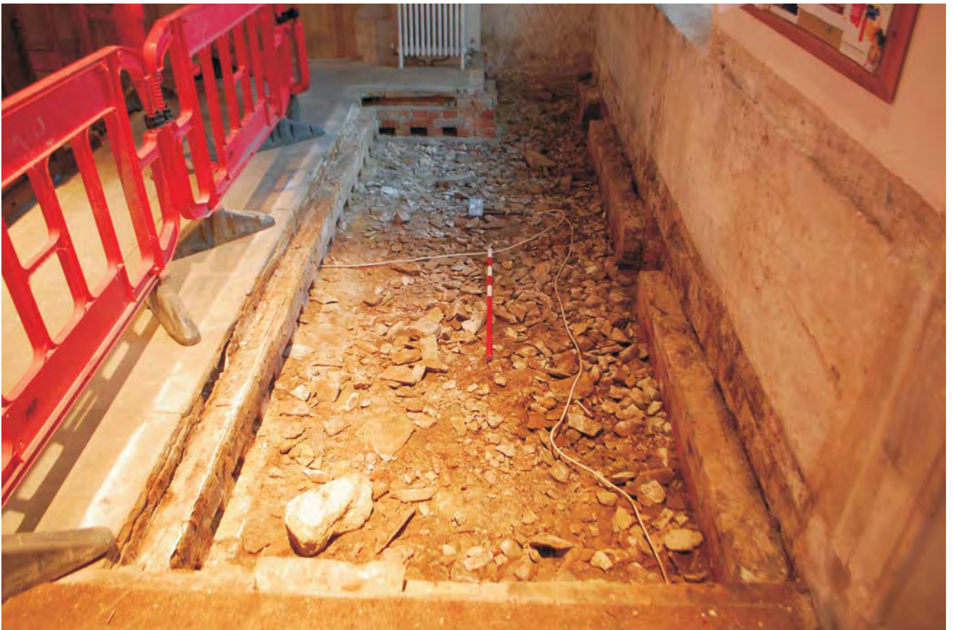
Plate 15. Interior view of Area D in St Mary's Church, Frittenden looking east showing brick dwarf walls to support timber pew floor and recent rubble infill ( note: small projecting spur area beside the radiator ).
