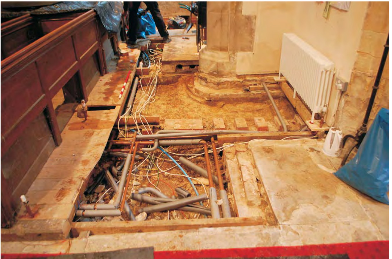
Plate 7. Interior view of St Mary's Church, Frittenden looking across Area A following the removal of the pews and timber flooring revealing the masonry foundation to the pier respond beneath ( note: brick dwarf walls to support timber pew floor ).
