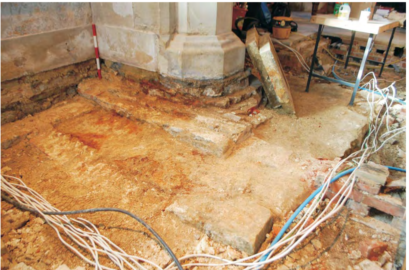
Plate 10. Interior view of St Mary's Church, Frittenden in Area A showing the upper extent to the masonry foundation to the pier respond following the removal of the brick dwarf walls ( note: hewn ashlar stone blocks forming the outer extent to the foundation ).
