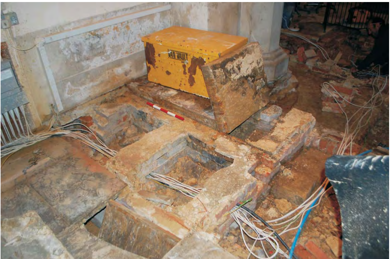
Plate 8. Interior view of St Mary's Church, Frittenden looking across Area A following the removal of the pews and timber flooring revealing the brick dwarf walls supporting the stone slab floor overlying the masonry foundation to the pier respond ( note: excessive brick support walls possibly to support internal stove? ).
