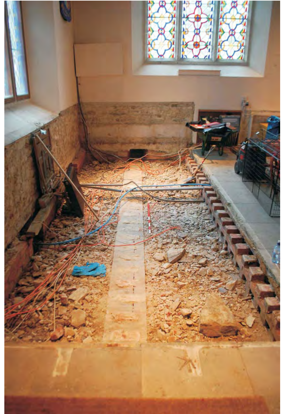
Plate 12. Interior view of Area C in St Mary's Church, Frittenden showing brick dwarf walls to support timber pew floor and recent rubble infill.
