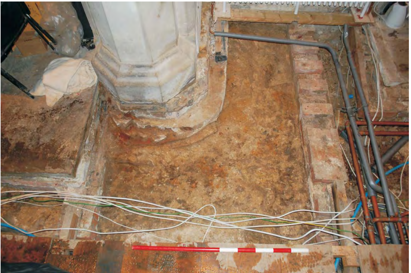
Plate 9. Interior view of St Mary's Church, Frittenden in Area A showing the upper extent to the masonry foundation to the pier respond ( note: layer of broken bricks beneath the moulded pier respond base ).
