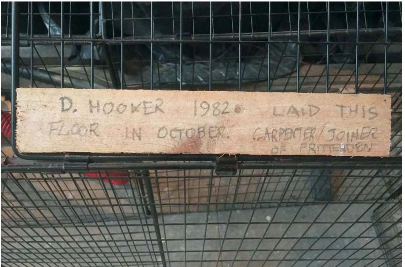
Plate 17. Image of a small timber off-cut discarded beneath the pew floor with inscription.
