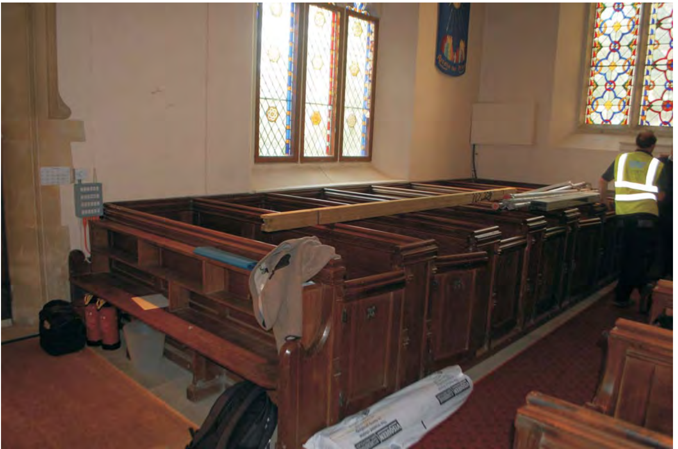
Plate 5. Interior view of St Mary's Church, Frittenden looking southwest across Area C prior to removing the pews and timber flooring.
