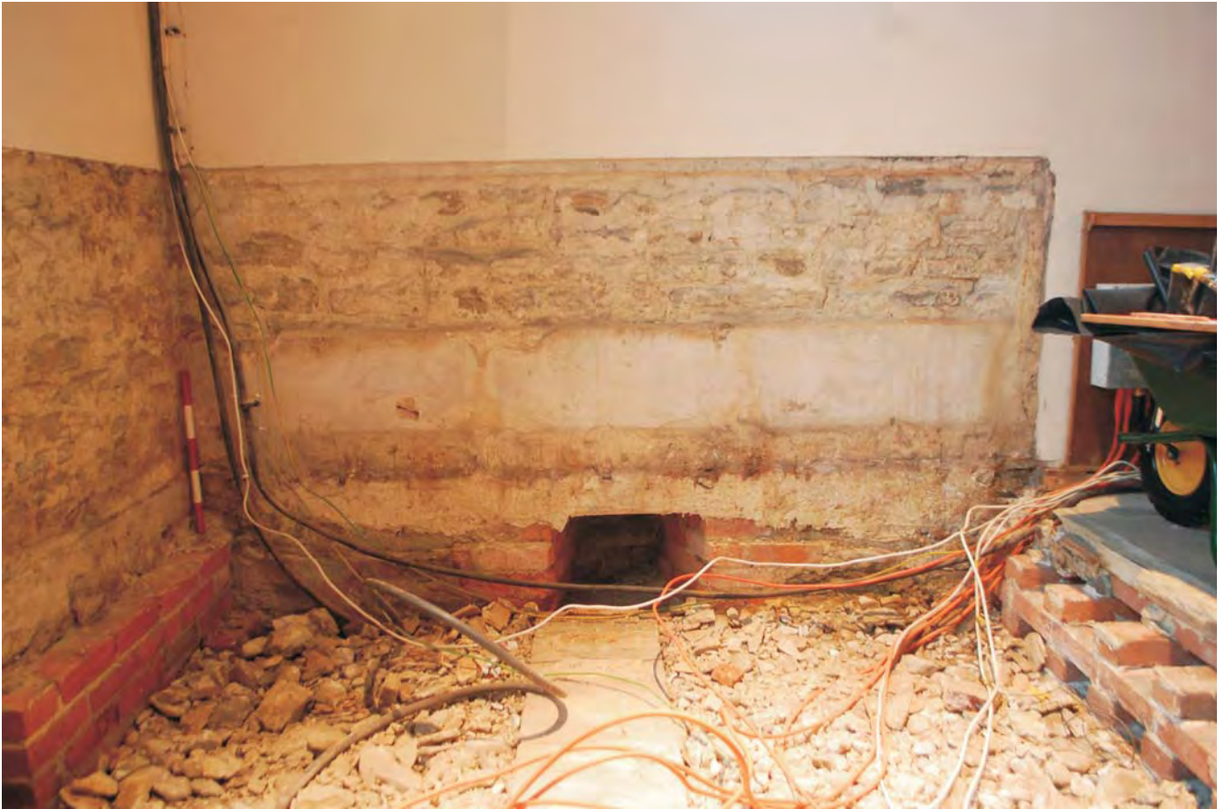
Plate 13. Interior view of Area C in St Mary's Church, Frittenden looking west showing the air vent opening through the base of the south aisle's west wall.
